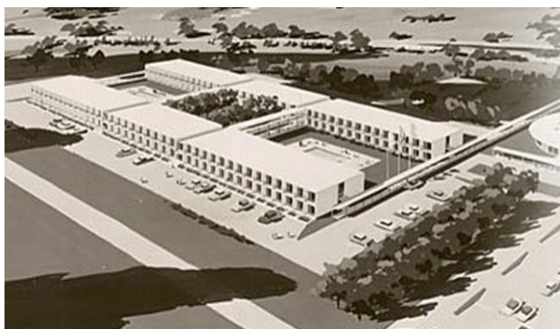
Figura 15 San Francisco Airport Hilton
